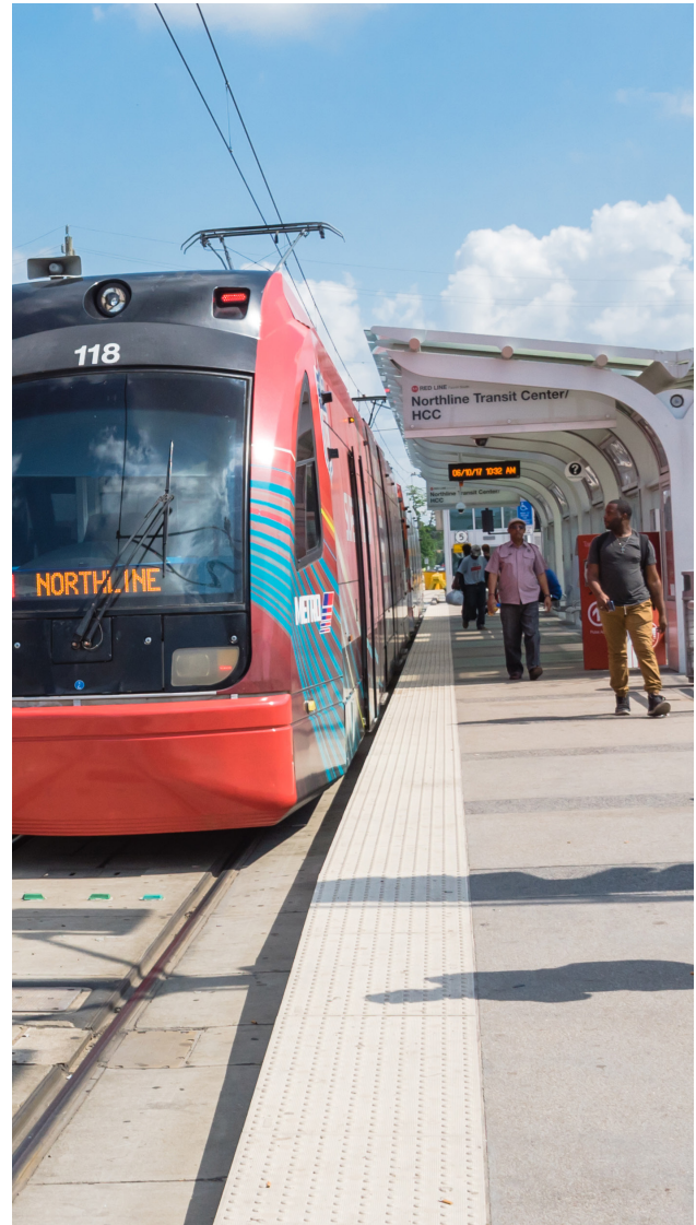
METRO's Red Line takes riders from the Northwest Transit Center to downtown in an average of 20 minutes.
